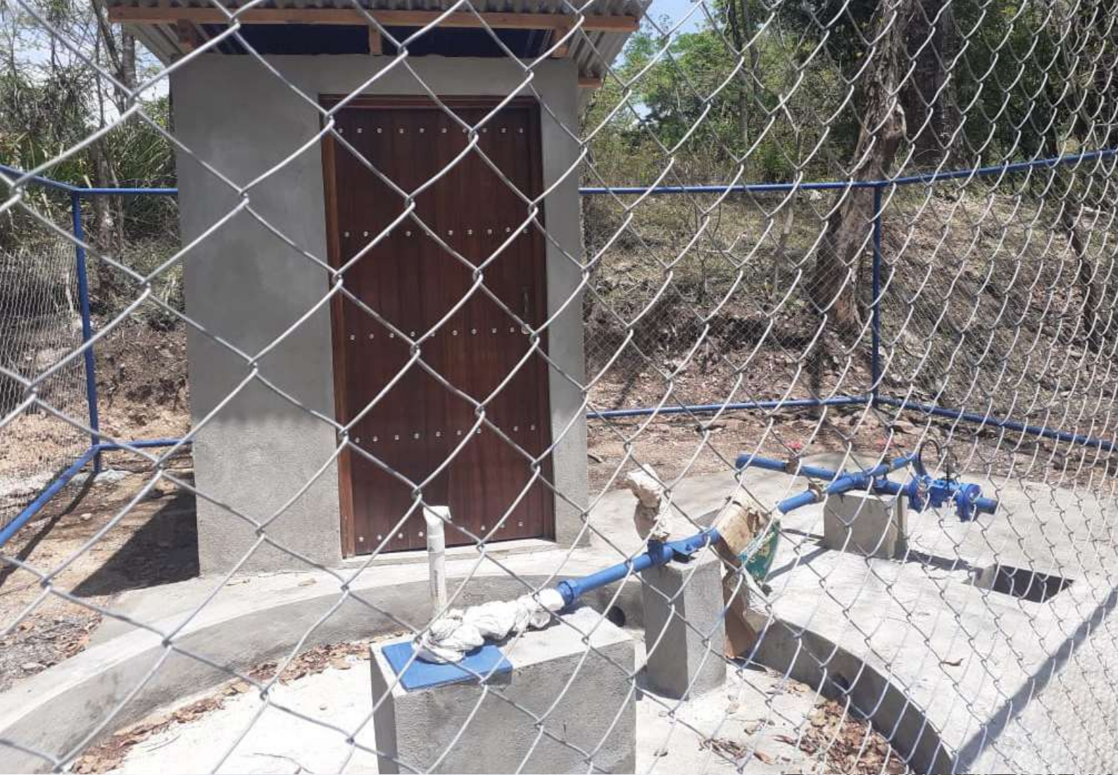
Completed pump house and distribution tank
