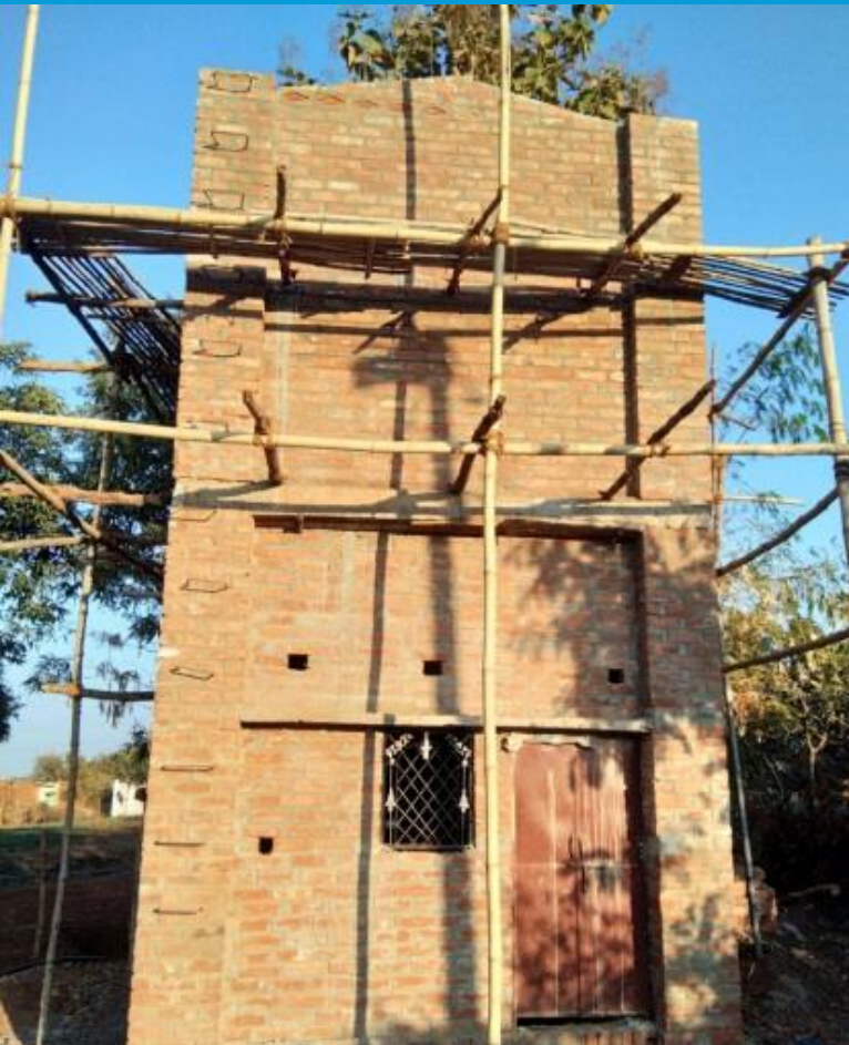
40,000 litre capacity elevated reservoir under construction
