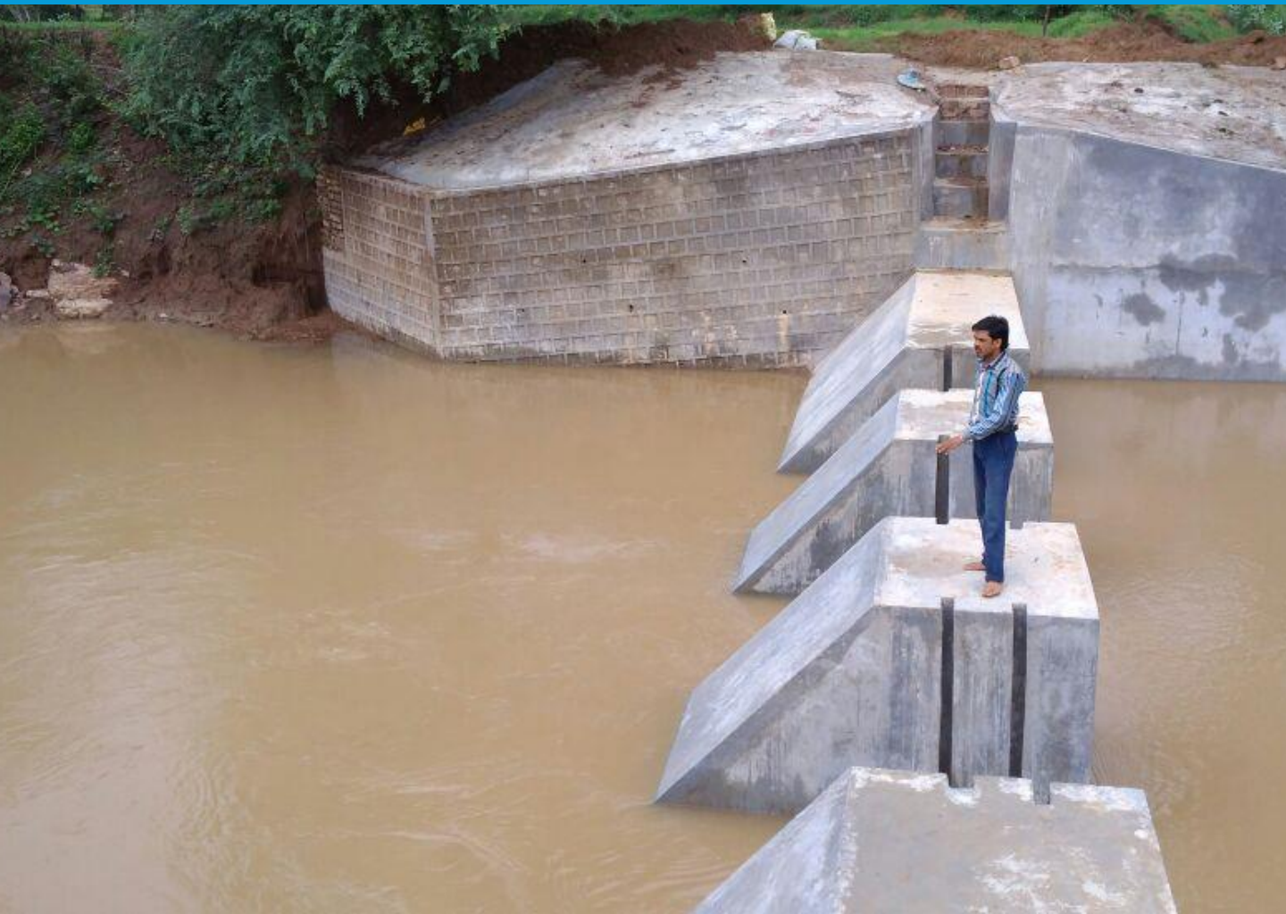
Renovated check dam
