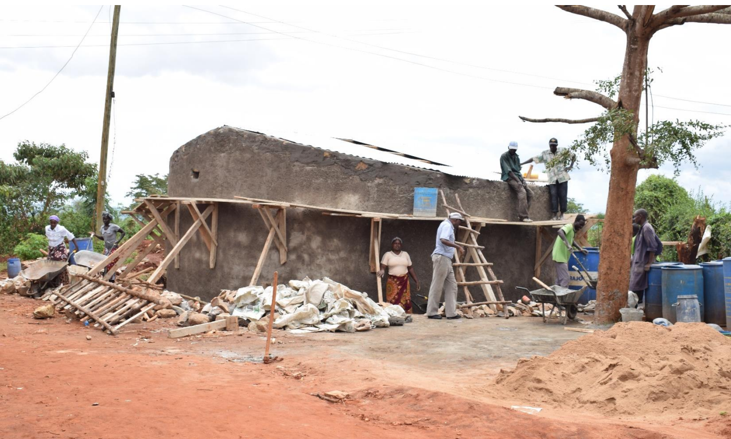
Mbukilye Ngukilye Widows Self Help Group working on the tank construction
